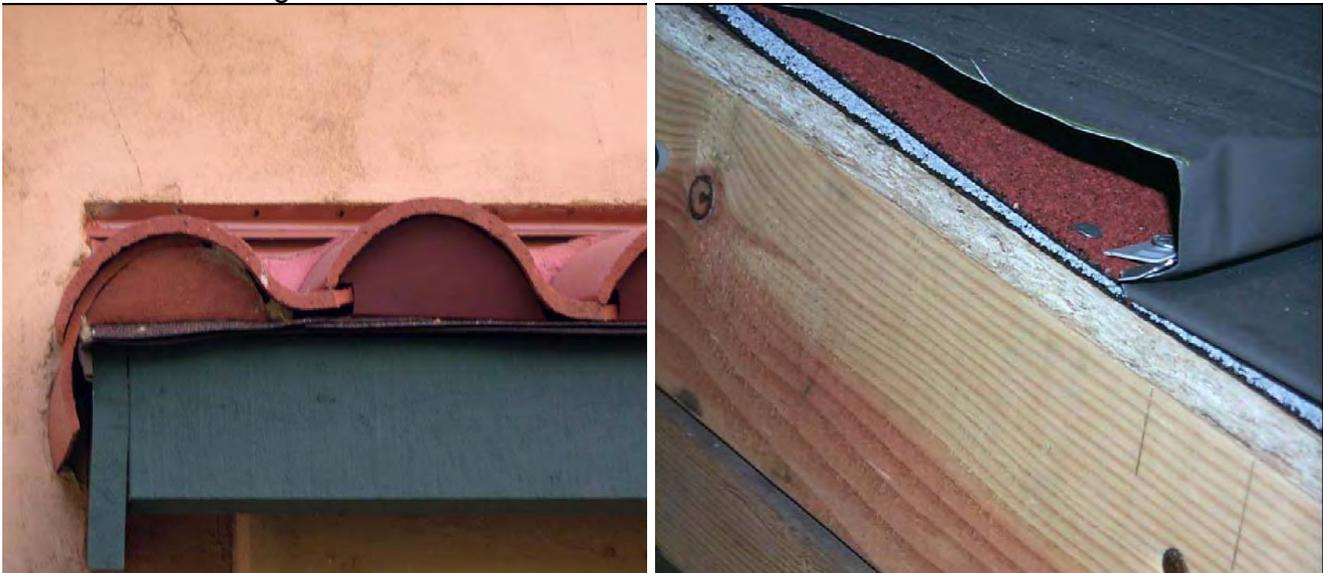
Cap provided to restrict intrusion of brands onto the roof deck. The other option is to provide one layer of No. 72 ASTM cap sheet installed over the combustible decking.
